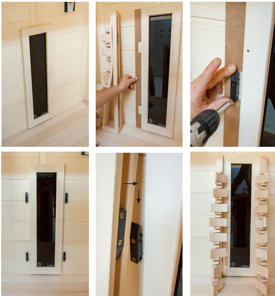
Fig. 29: Installing the backrests
