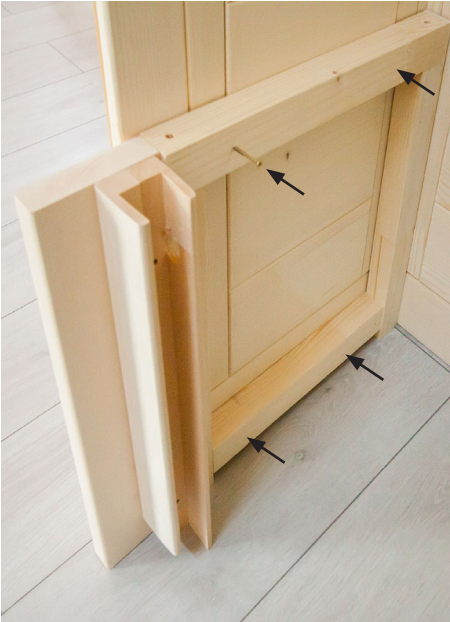
Fig. 18: Installing the bench supports
