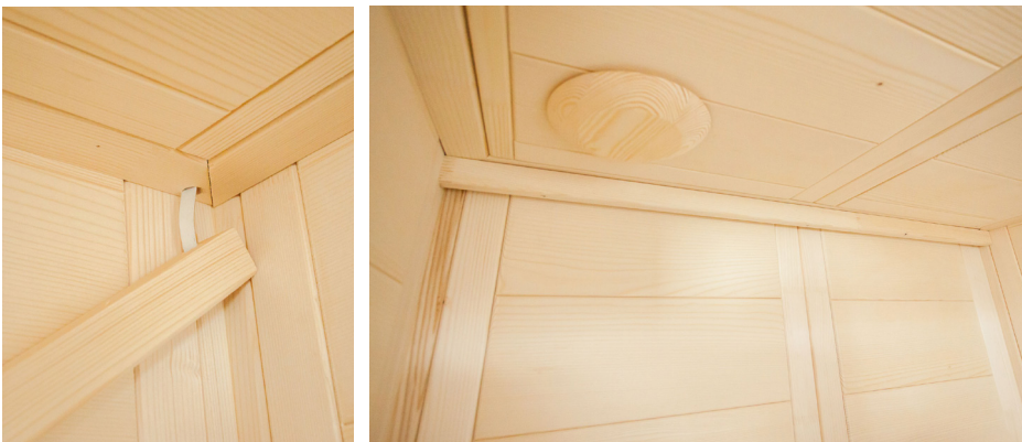
Fig. 24: Attaching the LED strip
