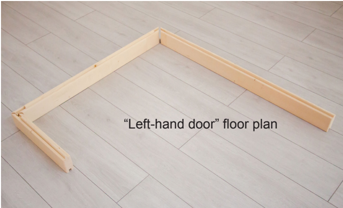
Fig. 1: Laying the three base frame elements
