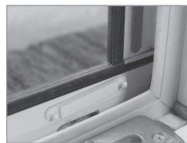
4. Place the magnetic holders (**2**) with the magnets onto the small metal plates which are attached to the window frame.
