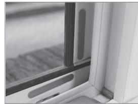
3. Attach the small metal plates (**3**) inside the window frame:
