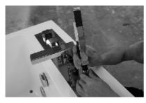
2. Put the shower head into the bathtub in right position as pic. Shows.
