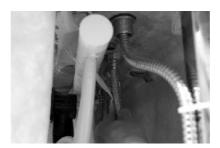
5. Distinguish the water pipes of faucet. Use spanner to screw the tie in.
