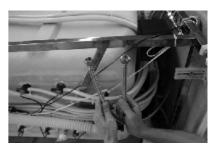
Connect the cold and hot water pipes.
