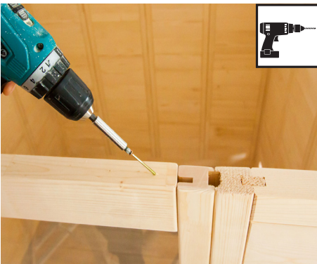
3 mm drill bit, 1 screw 4 x 70 mm
