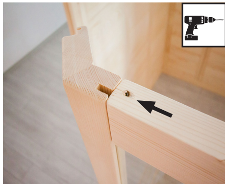
3 mm drill bit, 1 screw 4 x 70 mm
