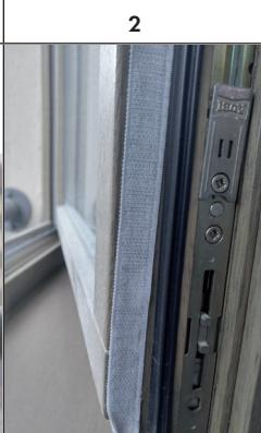
A close-up photograph showing the velcro strip attached to the window frame. The window is open to the right. |
