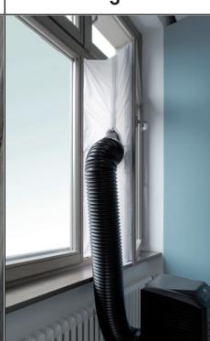
A wider photograph showing the window fully open. A black flexible plastic duct is connected to the bottom of the window frame, which is covered by the grey velcro seal. The room interior and a radiator are visible in the background. |
