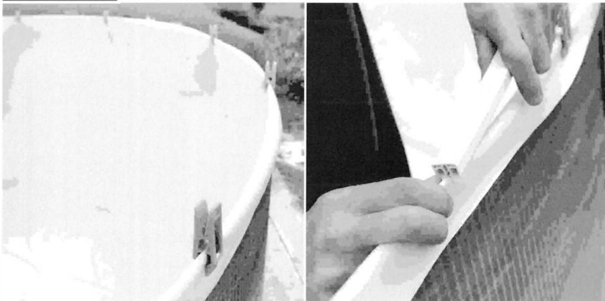
**EN** Note: Some references **HAVE NO FLEXIBLE OVERLAP** (SF) on the liner side. The liner must be hung by folding it over the wallplate so that an even 3-4 cm overlap is left.
