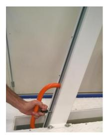
Loosen the floor fastening.
