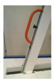
The heights are shown on the shaft next to the bracket for the height adjustment.
