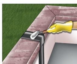
5. Press down the tape (using a roller or similar device). Make sure the tape is fully sealed to the surface.
