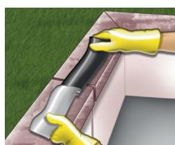
4. Remove the protective film (on one or both sides, depending on the type) from the tape and place the tape on the element to be repaired.
